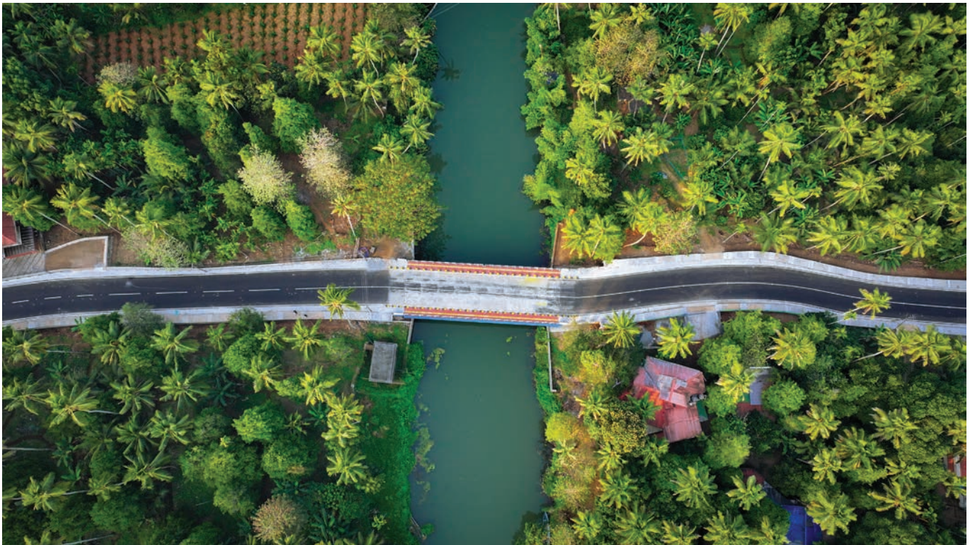
Sreedhari bridge across Manali river in Thrissur District
