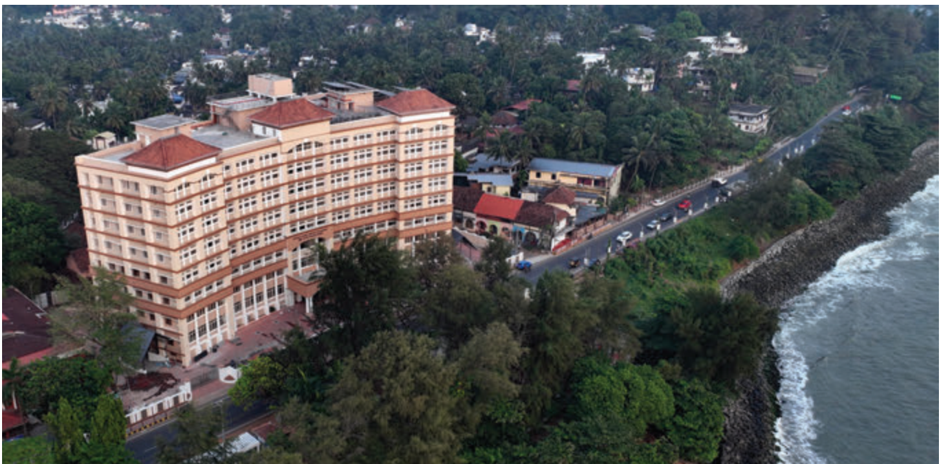
Thalassery Court Complex
