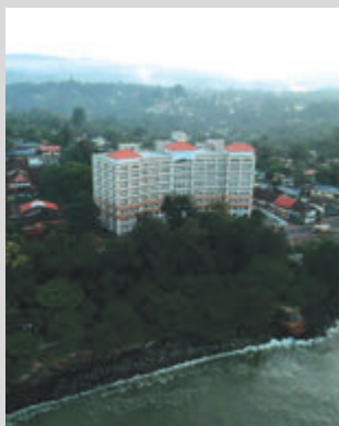
Court Complex - Thalassery Courtesy : Greeshma R Pillai, Project Engineer, Project Appraisal Division
