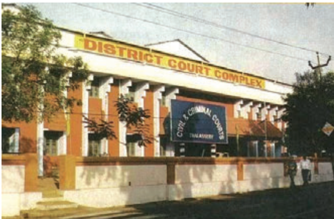
Thalassery Court Complex- (Old Building)
