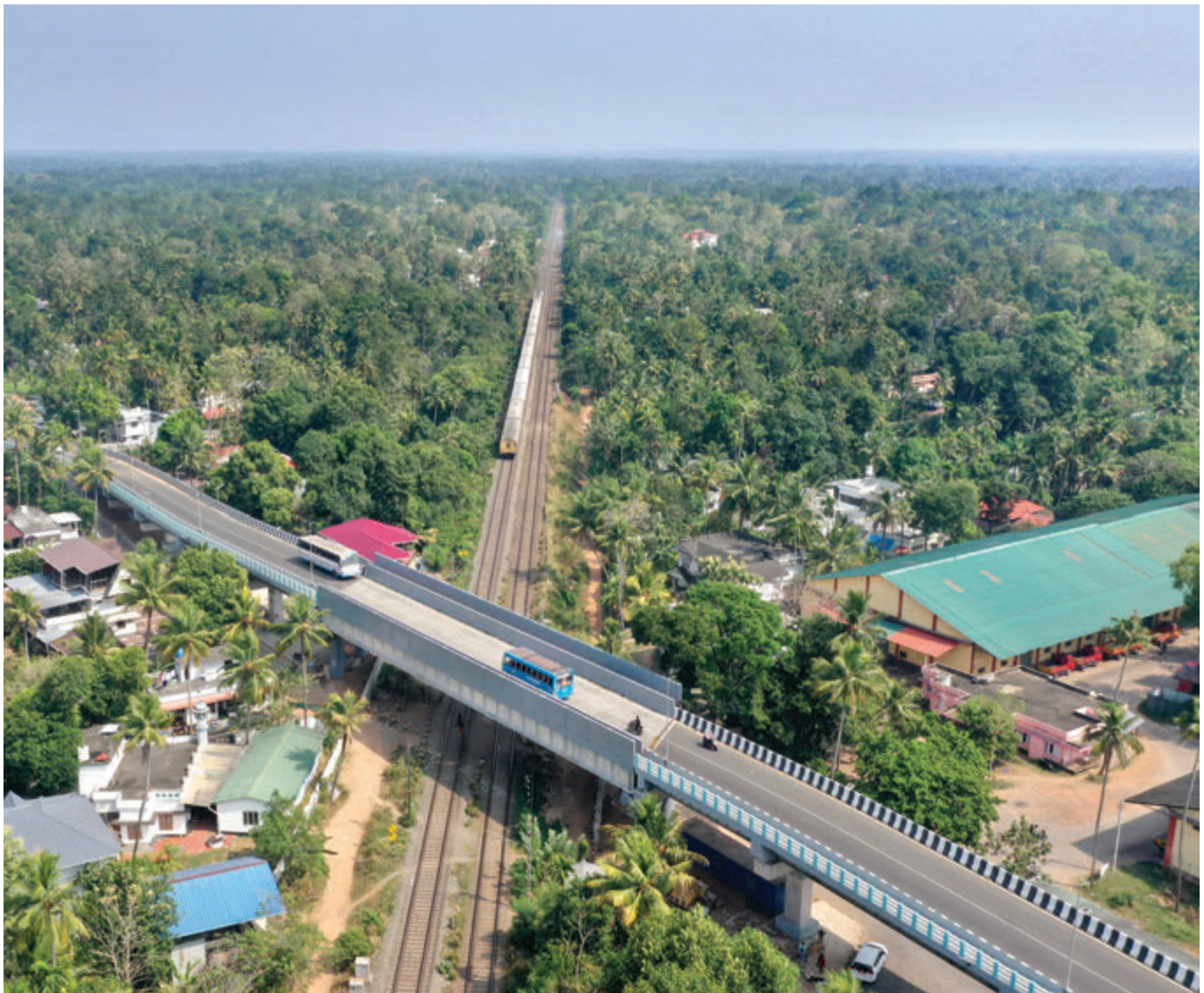
Maliyekal Railway Over Bridge
