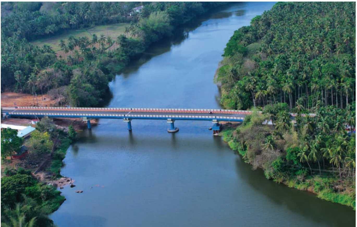
Kondazhy Kuthampully bridge
