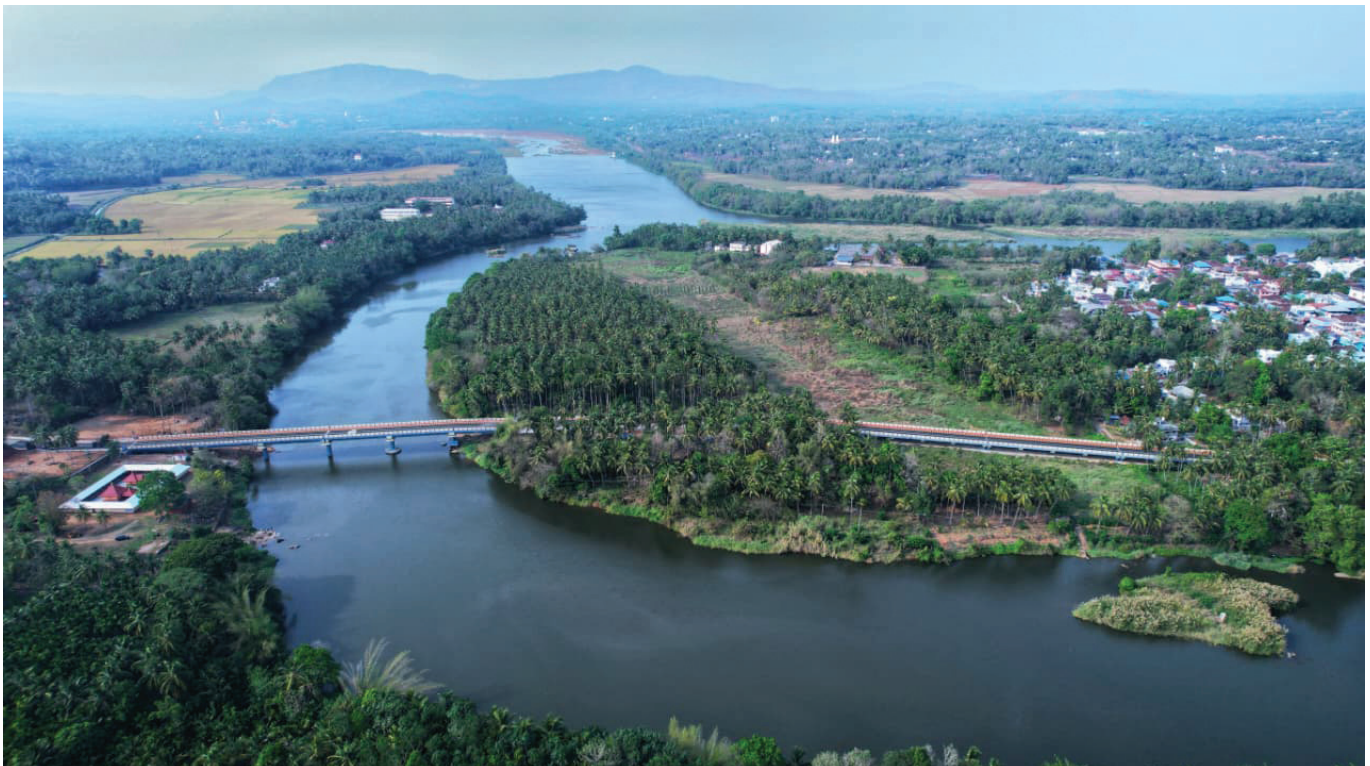
Kondazhy Kuthampully bridge
