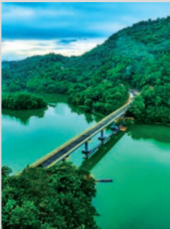
Amboori Kumbichal Kadavu bridge Courtesy : Mohammed Irshad R Senior Inspection Engineer
