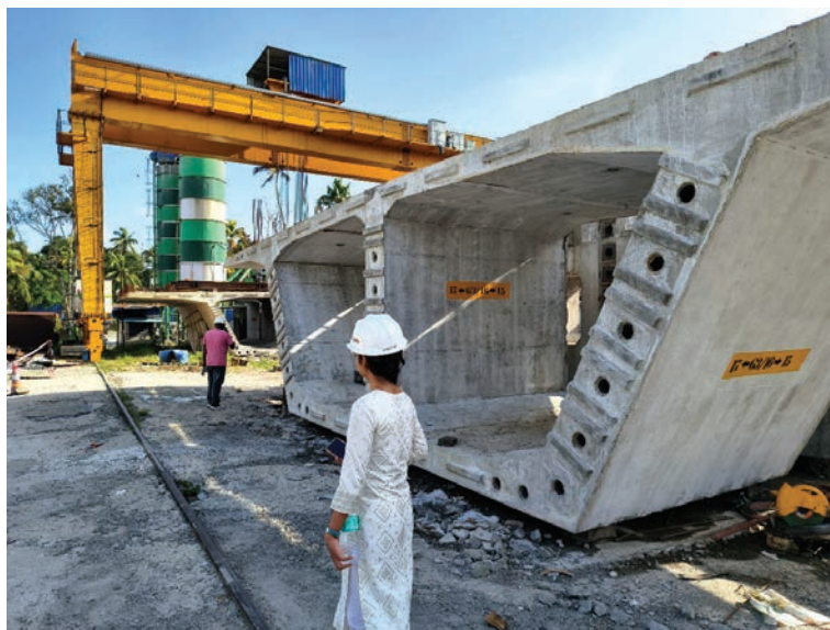
A cast segment with shear keys visible at end
