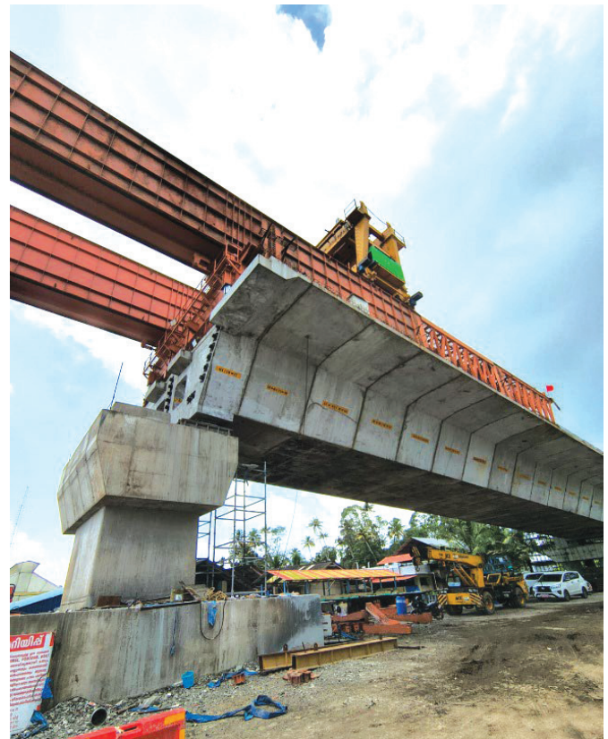
Auto-Launch method in Azhikode-Munambam Bridge
