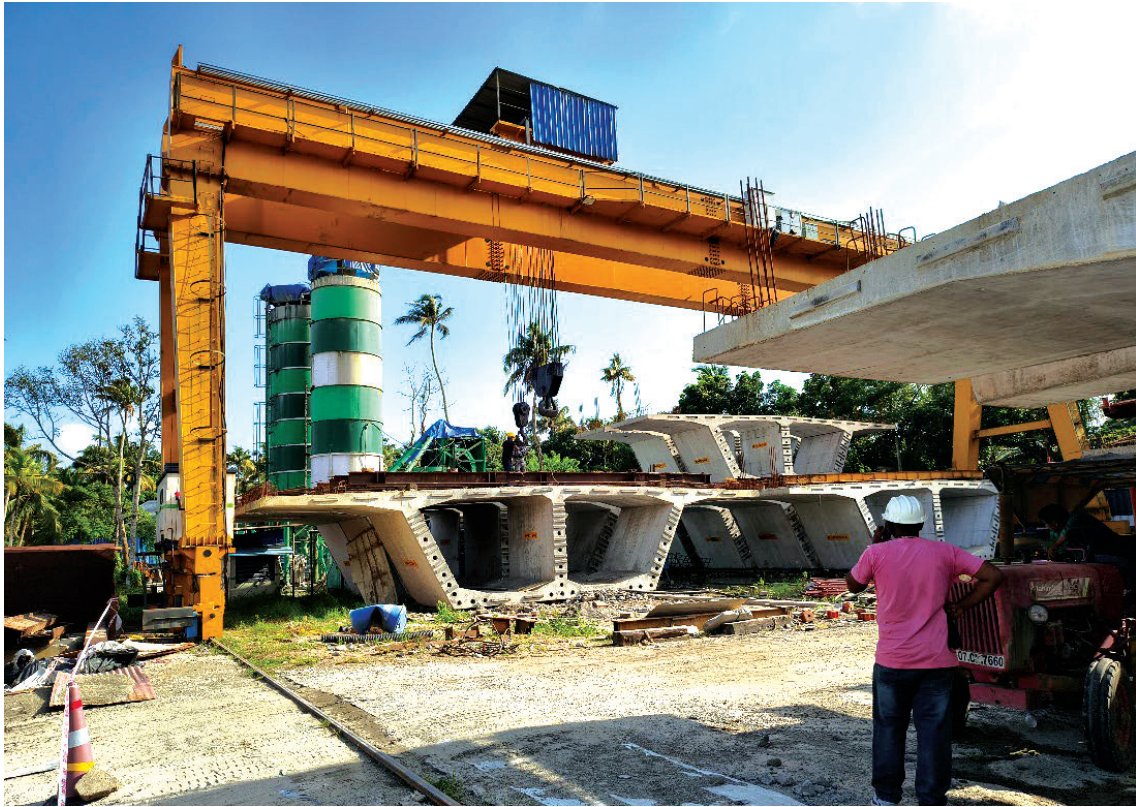
Cast segments stacked at the stacking yard
