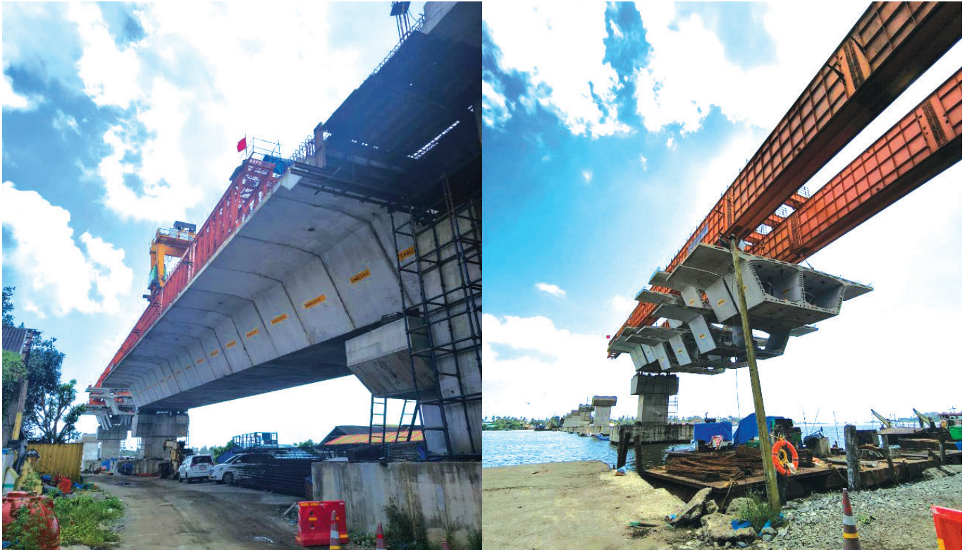
Completed Span and Matching of the Subsequent Span
