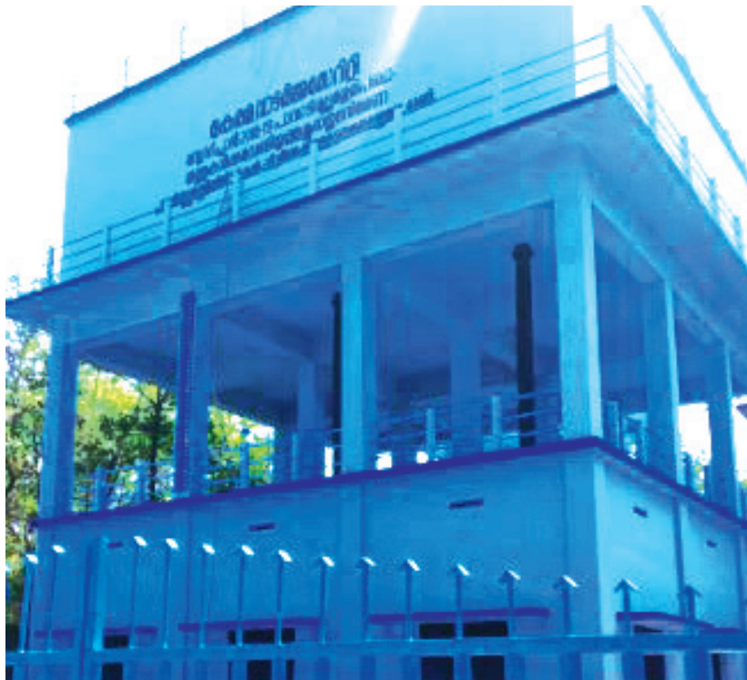
Over Head Service Reservoir
