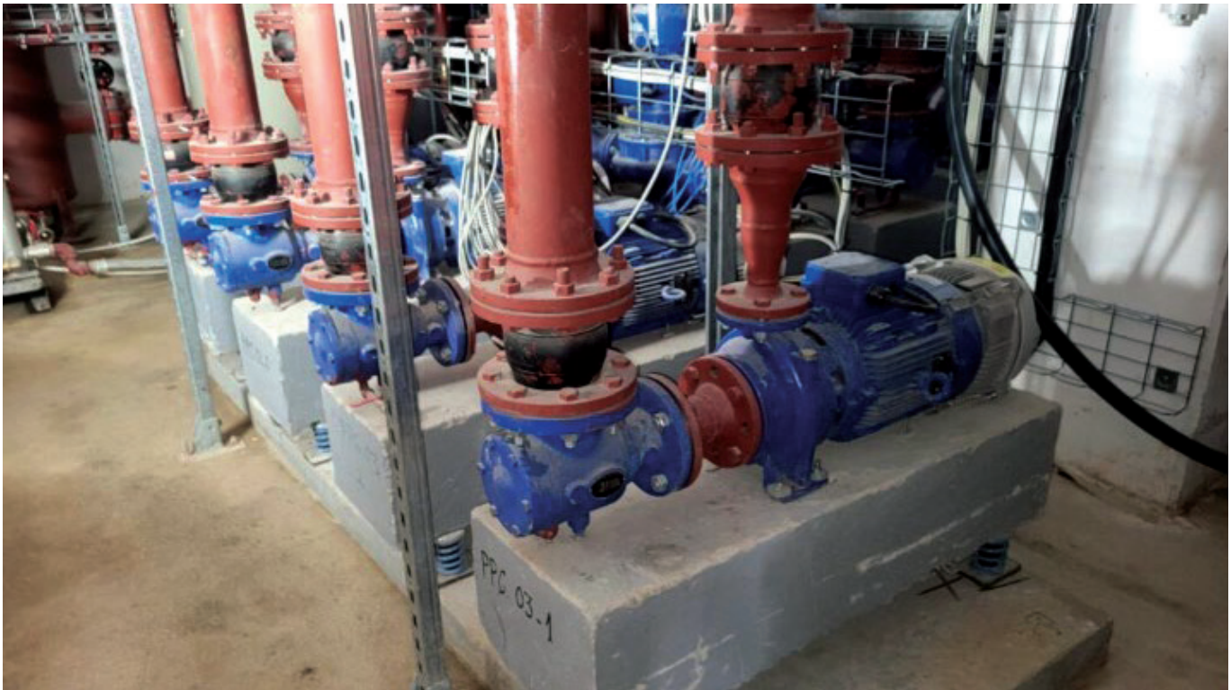
Fig 2: Suction Diffuser installation on suction side of pump
